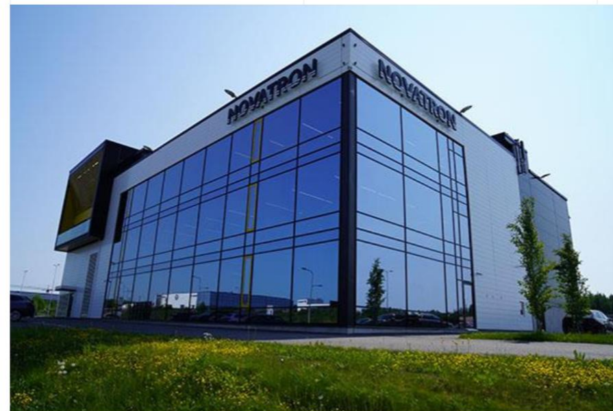
Technology Center in Pirkkala, Finland
